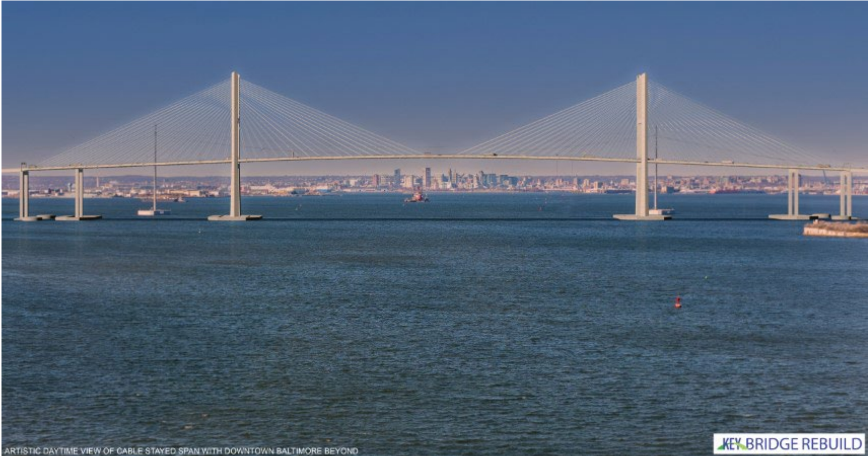
ARTISTIC DAYTIME VIEW OF CABLE STAYED SPAN WITH DOWNTOWN BALTIMORE BEYOND
