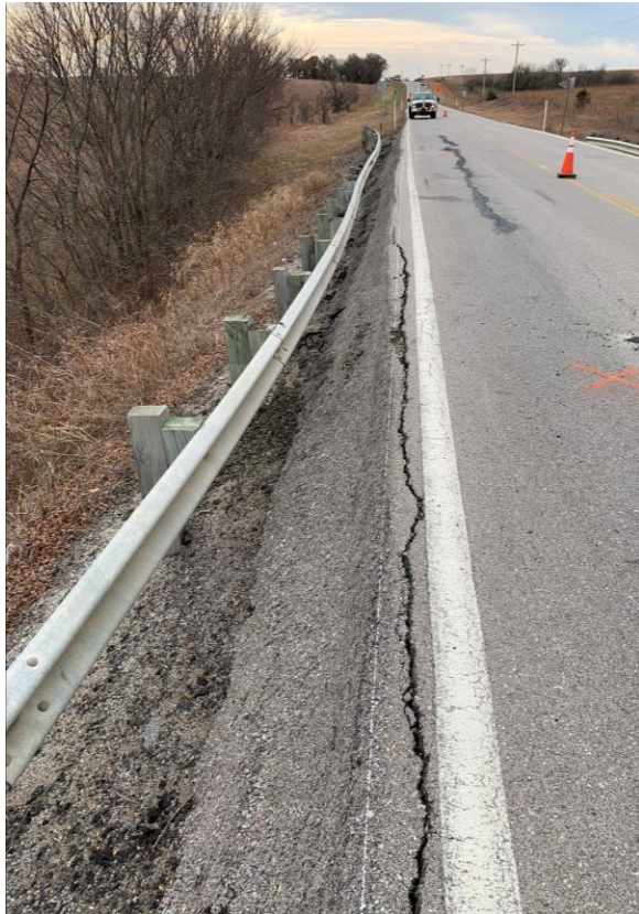
Cracking/Settling of Pavement
