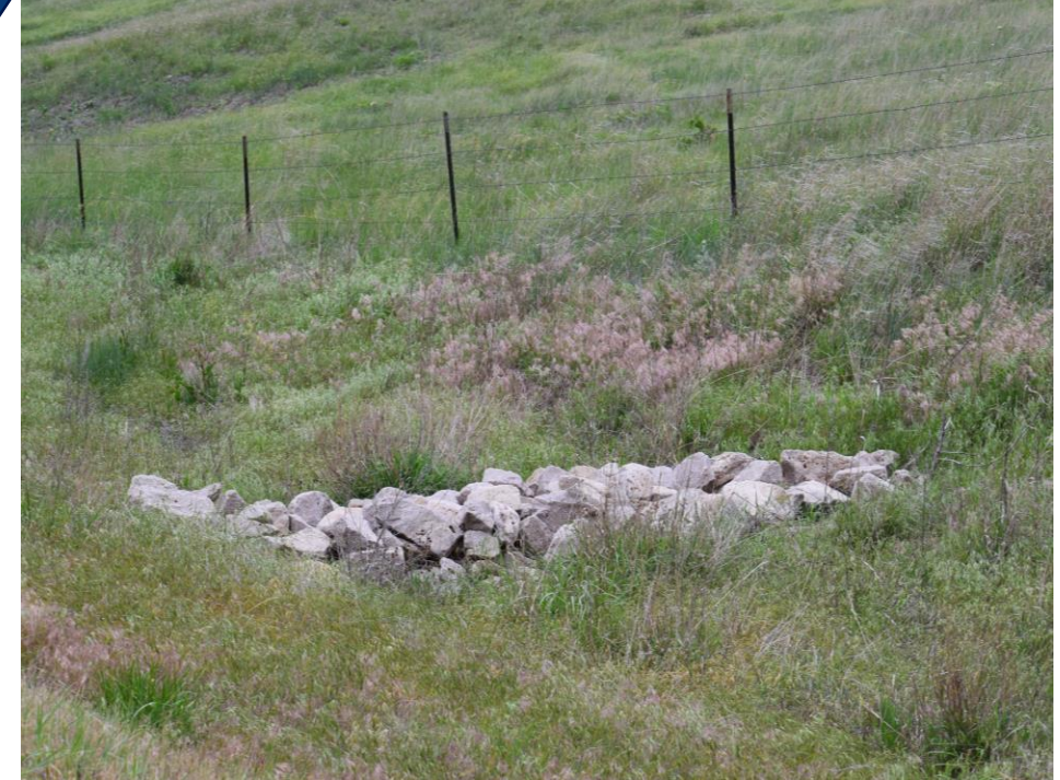
Erosion Control Barrier
