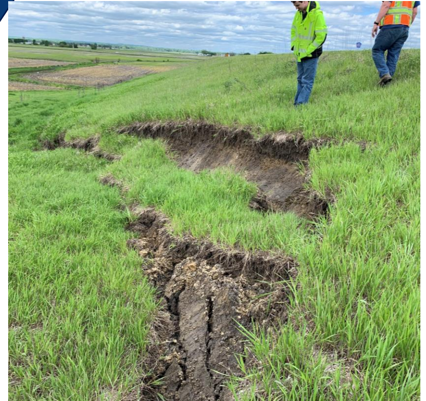
Slickensides and Cracking along scarps
