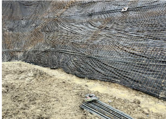
Step 4: Place and tie continuous waler bar.
