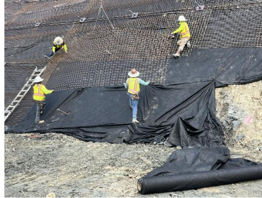
Step 2: Place wire mesh sheet.
