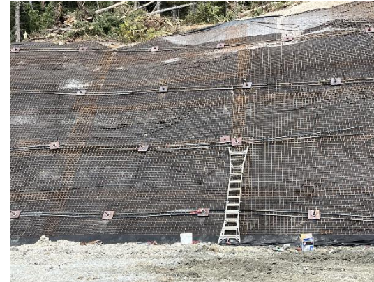
Step 5: Place bearing plate, beveled washer, and collar nut.
