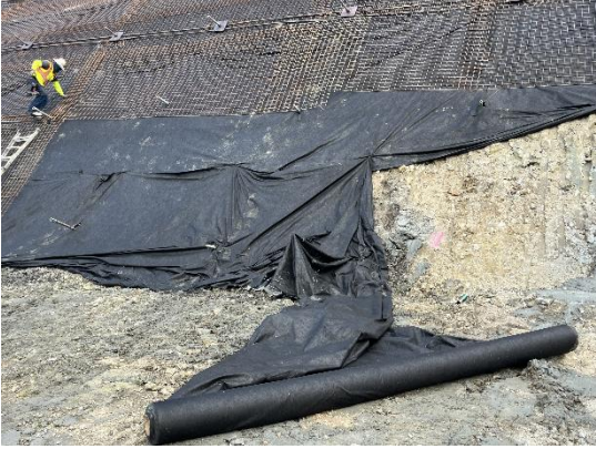
Step 1: Place and secure geotextile.
