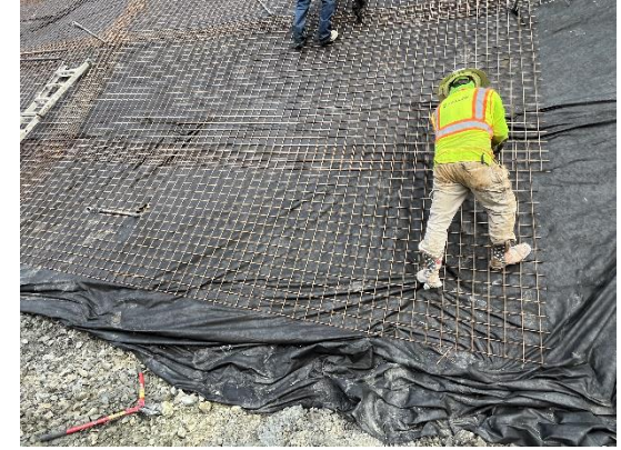
Step 3: Tie wire mesh properly.
