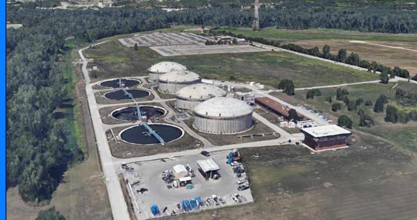
Blue River WWTP, Kansas City
