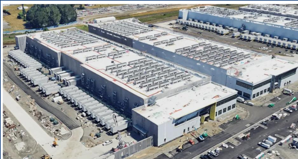
A recent Data Center just completed along NE Huffman Drive, just West of Brookwood. Note the backup generators and roof-mounted AC Units.
