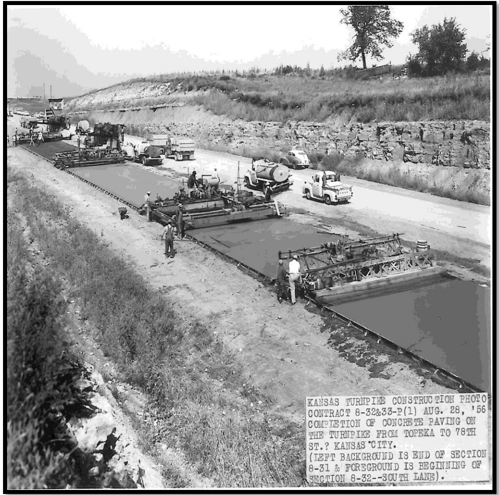
Concrete Pavement – MM 177 to MM 236
